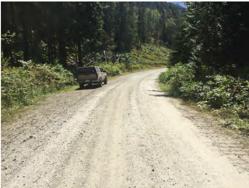
Left Approach Facing Away From Culvert
