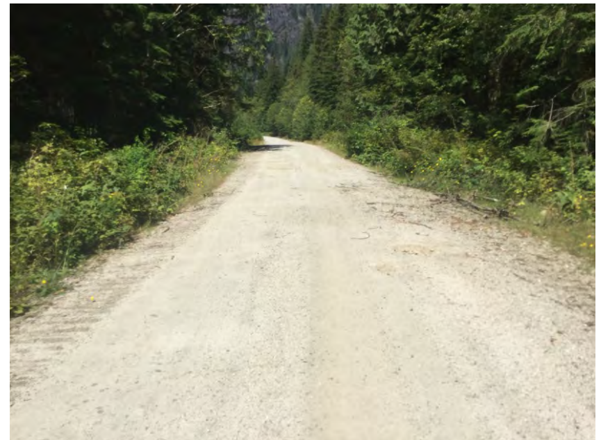
Right Approach Facing Away From Culvert
