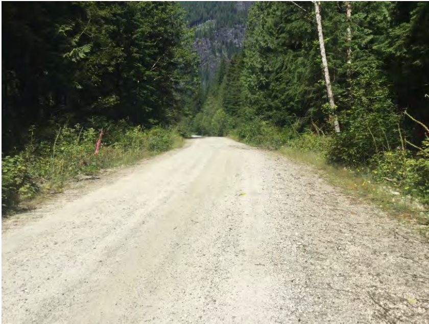
Left Approach Facing Culvert
