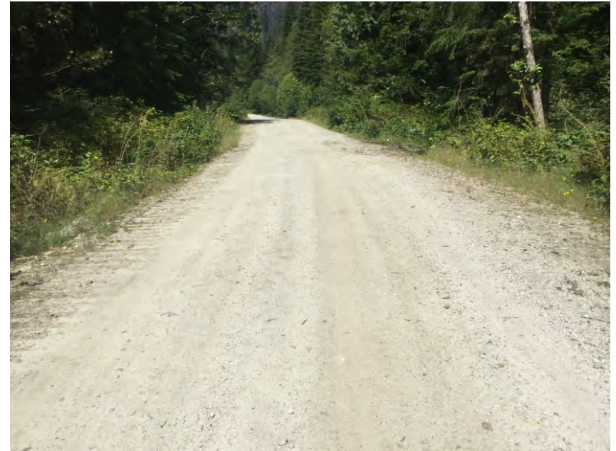
Roadway Over Culvert
