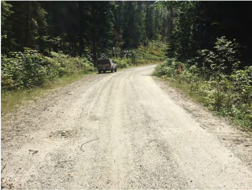
Right Approach Facing Culvert
